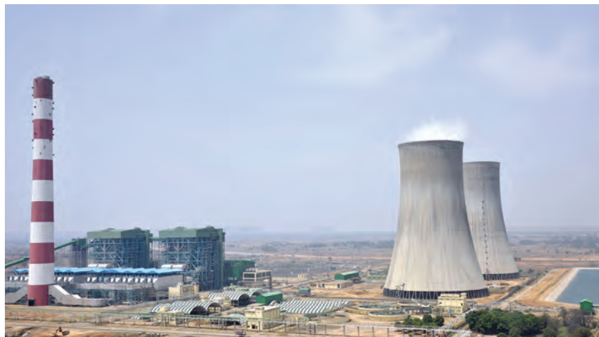
CLEANER PLANT In India, this 1,300-MW supercritical coal plant was commissioned in 2015.
