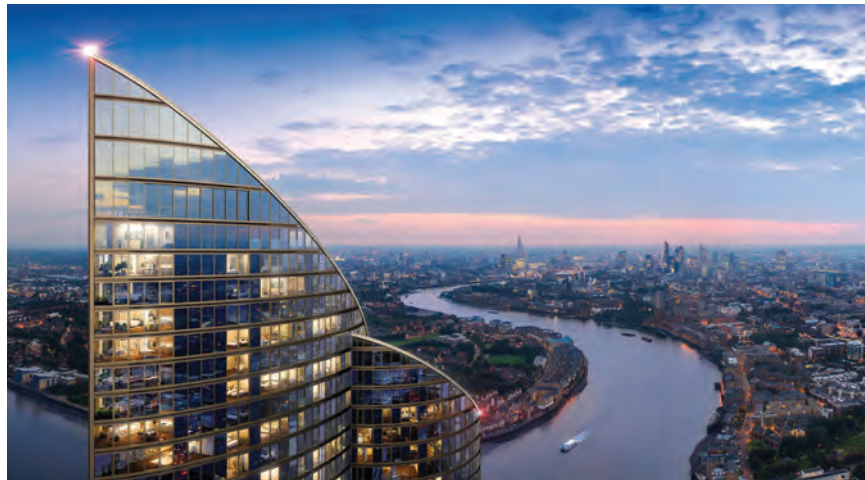
NEW DIGS AECOM is building the 67-story Spire London residential tower, set to be the tallest in western Europe.
