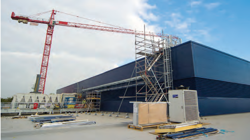
INCREMENTAL EXPANSION Fluor expanded the Solvay adhesives plant in Wrexham, Wales.
