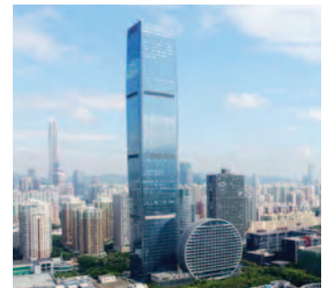
2016 Tallest #10: Shenzhen CFC Changfu Centre, Shenzhen, 304 meters © Cheng Chen
