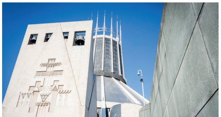
Heritage: Purcell is working on the repair of Liverpool Met Cathedral.
